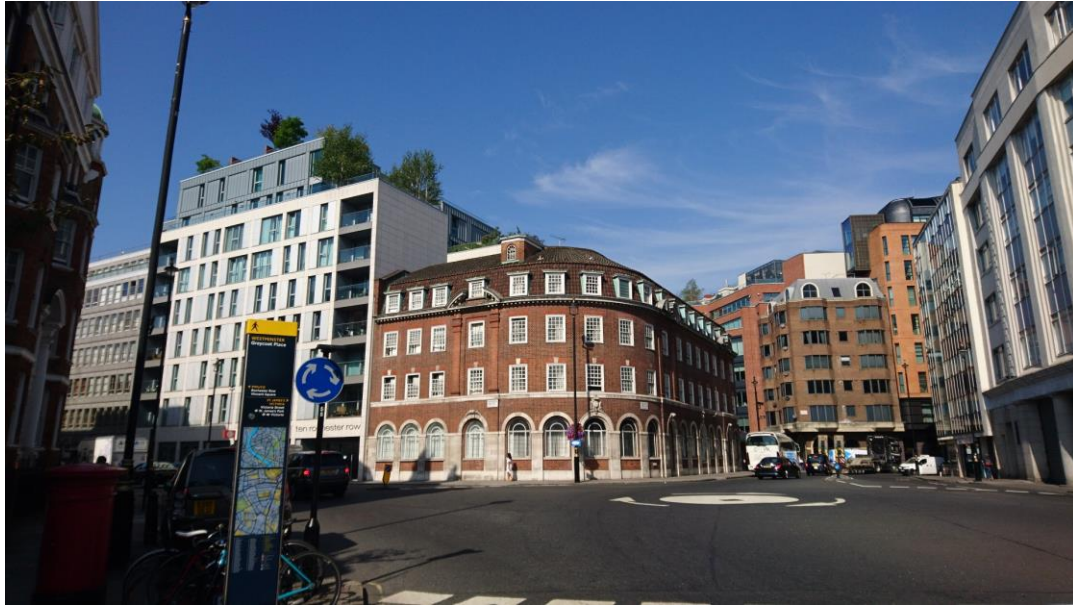
Townsend House – view from Greycoat Place across to Rochester Row
